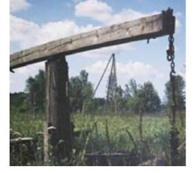
**BEAM AND THREE-POLE RIG** A pumpblock, the pioneer precursor to the pumpjack, frames one of Ontario's last original three-pole derricks. The derricks were used with a team of horses to raise and lower pipe for repairs and maintenance. Credit: *Earle Gray*
