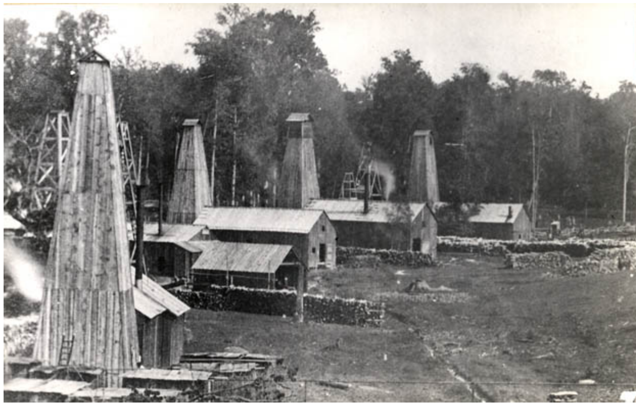
Drilling rigs in the Petrolia oil field, southwestern Ontario, in the 1870's. The rigs were sheltered to protect drillers from winter snow and summer rain. Photo courtesy Lambton County Museums.
